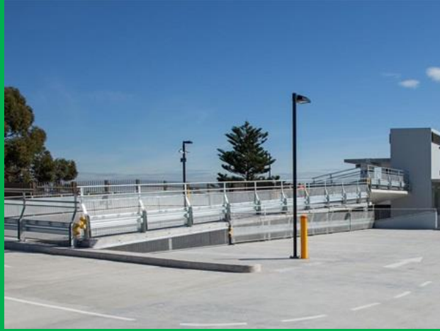
Padstow Commuter Car Park
