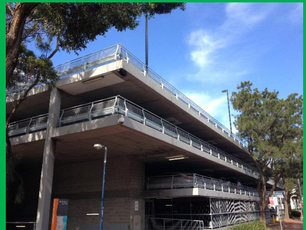
Wollongong Council Car Park Upgrade
