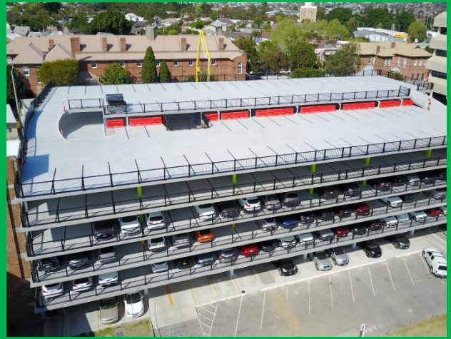
Newcastle Civic Car Park
